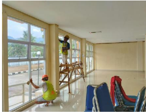
Pek. Pengecatan Interior
