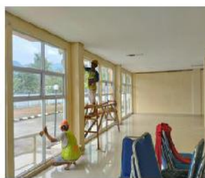
Pek. Pengecatan Interior
